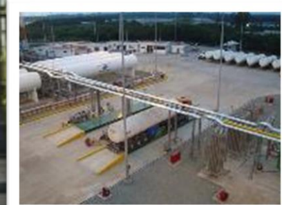
2015-Liquefaction: First plant 200 Tn/day in Equador
