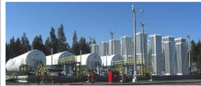
2011-TLF: First TLF in South America to supply the biggest PSR: 25.000 Nm 3 /h at 70 bar
