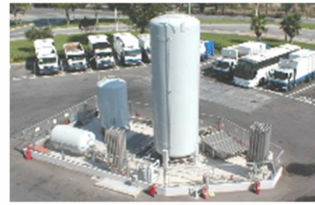
1999-CESPA BCN: First LNG Station to fill 25 MAN Trucks daily without pumps.
