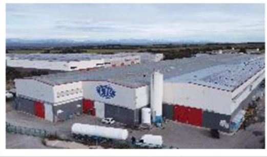
2018: New Facilities in Fonolleras
